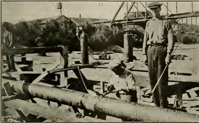
MAKING A FINAL WELD ON 100-FOOT SECTIONS OF PIPE IN MID-STREAM.
